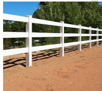
Post and rail fencing Supplier: Local contractor
