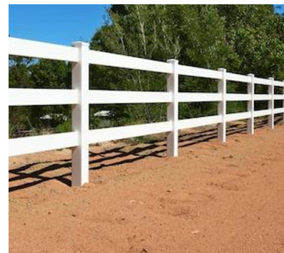
Post and rail fencing Supplier: Local contractor
