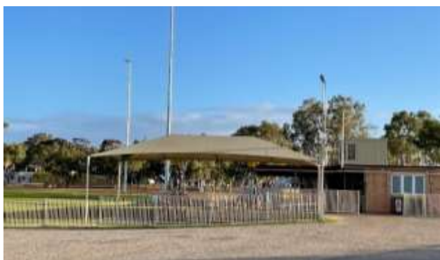
Pavilion with shelter (northern end) new LED lighting
