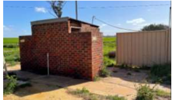
Public toilet block
