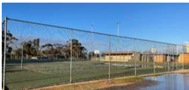
Courts subject to flooding – drainage poor
