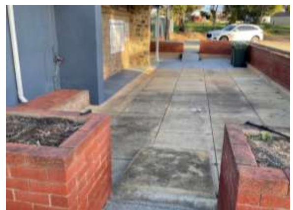
Ramped access at entry
