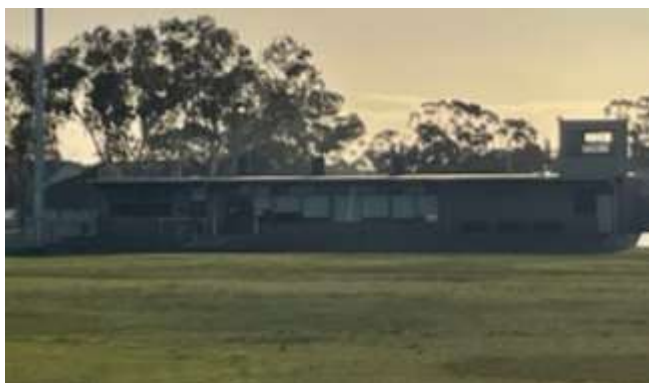
Sporting pavilion – community building & shelter
