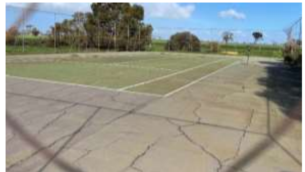
Surface cracking
