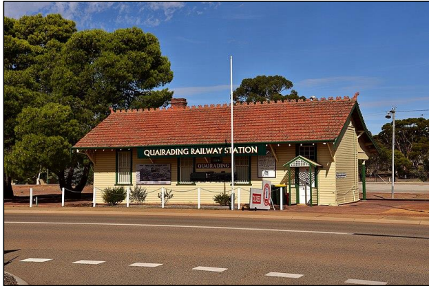
Railway Station Place listed on the Quairading MHI
